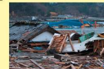
The earthquake caused a huge tsunami, which flooded the affected area
